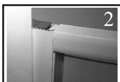
2. Fit channel cap-push fit.
