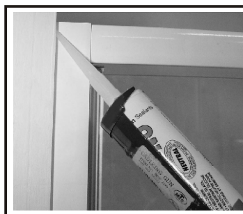
Silicone seal wallposts to wall on inside and outside
