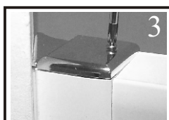
3. Fit top cap screw fix-no.4x10mm csk screws.
